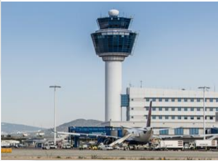
ATHENS INTERNATIONAL AIRPORT
